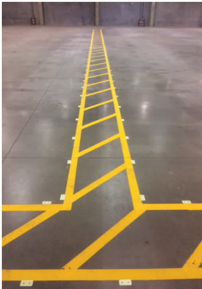
G7 Solaris Path Markers placed on outside of painted path
