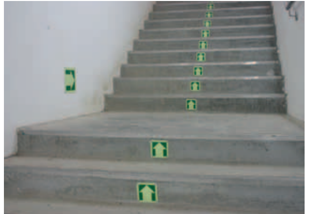
Marine Coastal Expressway - Singapore
