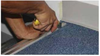
Packer in image is aluminium, but timber is also suitable
